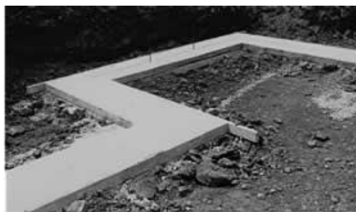
Concrete "Spread" Footing
